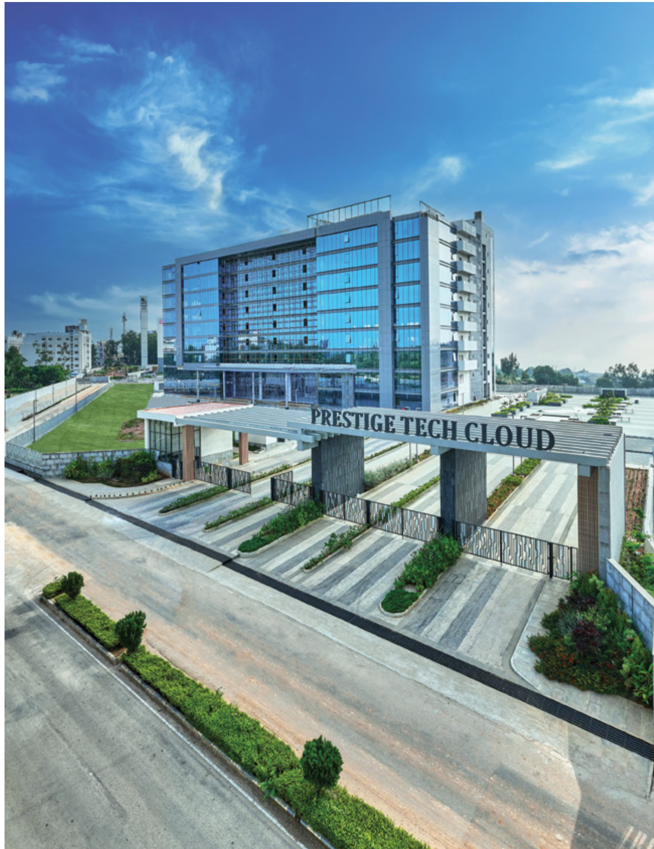
Prestige Tech Cloud is a world-class tech campus, located close to Kempegowda International Airport in Bengaluru. With contemporary clean lined aesthetics and large floor plates, it has ample open landscaped areas and congregational spaces.
