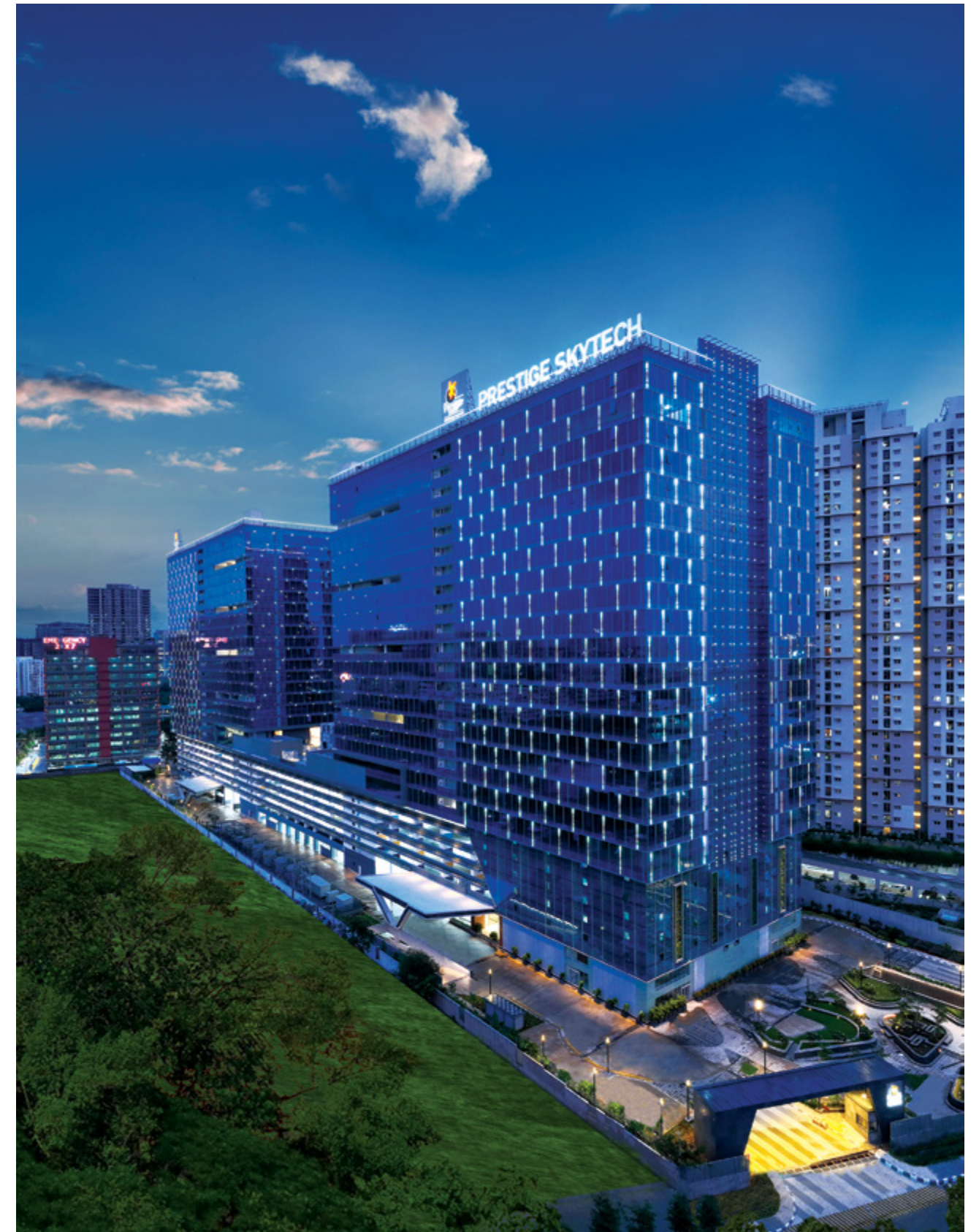
Prestige Skytech is an outstanding commercial office building in Karapakkam, Chennai that features contemporary design, state-of-the-art technologies and is home to major blue chip corporates and MNCs.
